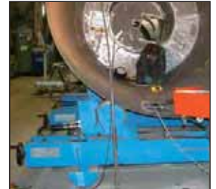
The operator adjusts the position of the can for tack welding via the remote control of the fit up rotators
